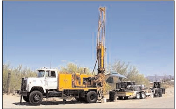
Drilling Rig at Tyson Wash Site.
