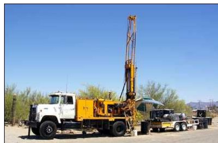
Drill Rig at Tyson Wash Site
