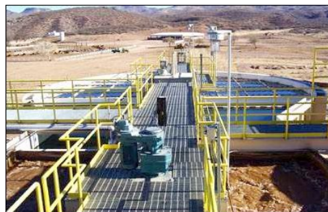
Overview of Water Treatment Plant at Lower Pinal Creek
