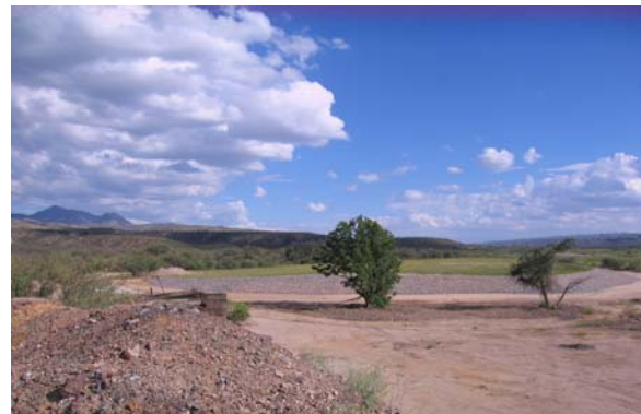
Completed Erosion Protection and Clean Cap on Upstream Tailings Pile
