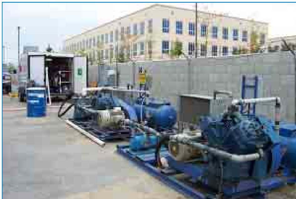
Figure 2: Soil Vapor Extraction System (SVE)
