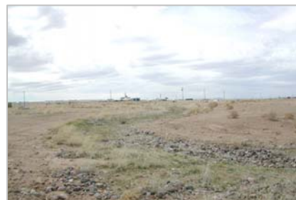
View of Landfill across Capped Area along Surface Drainage Channel
