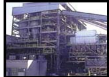
11-Story Oxygen Flash Smelting Furnace in Hayden
