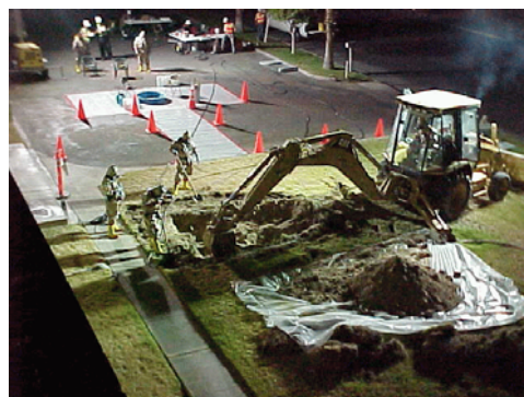
Uncovering a Septic System at the Houston Facility
