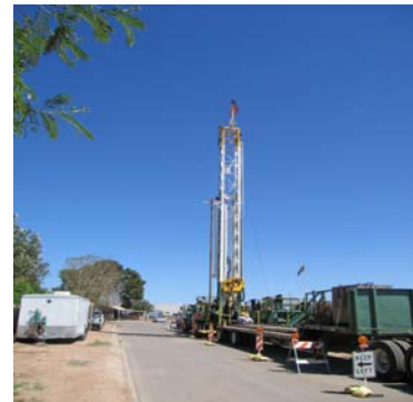
Installation of Monitoring Well
