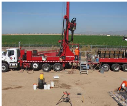
Drywell Investigation on the Unidynamics Facility
