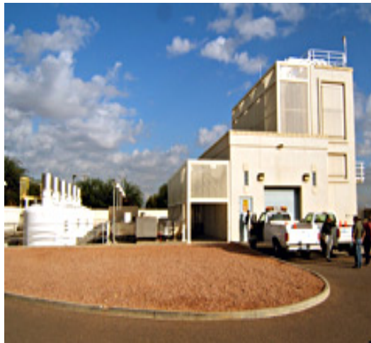
Central Groundwater Treatment Facility
