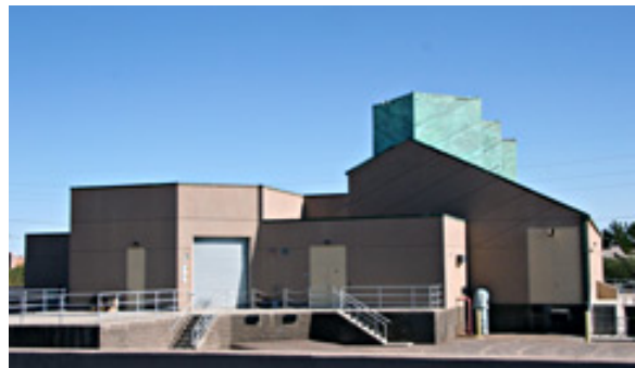
Miller Road Treatment Facility
