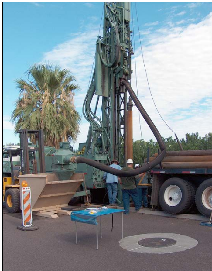
Monitoring Well Drilling.
