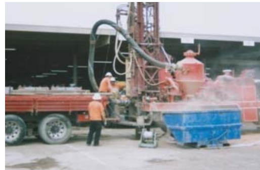
A Drilling Rig Installing a Monitor Well
