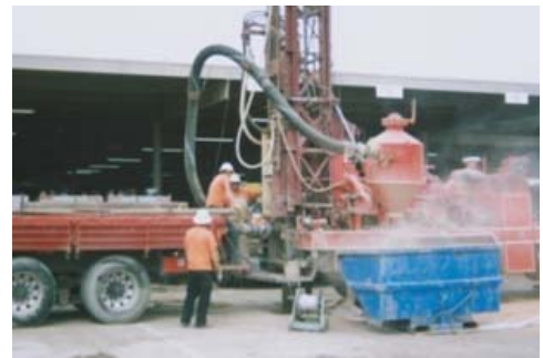
A Drilling Rig Installing a Monitor Well
