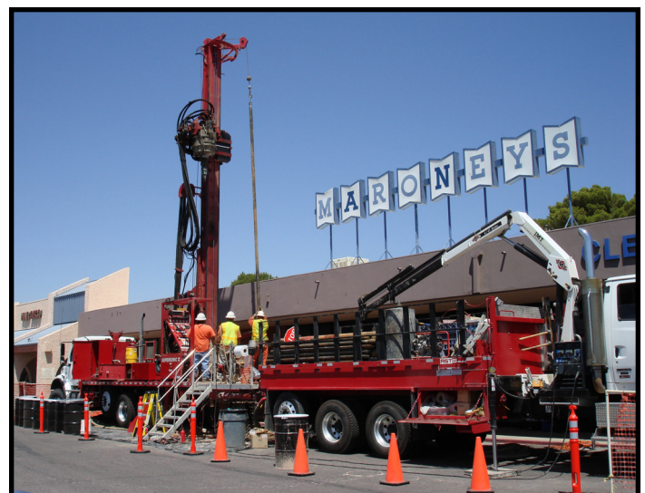
Well installation at the site.
