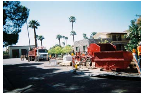
Drilling of off-site monitor well
